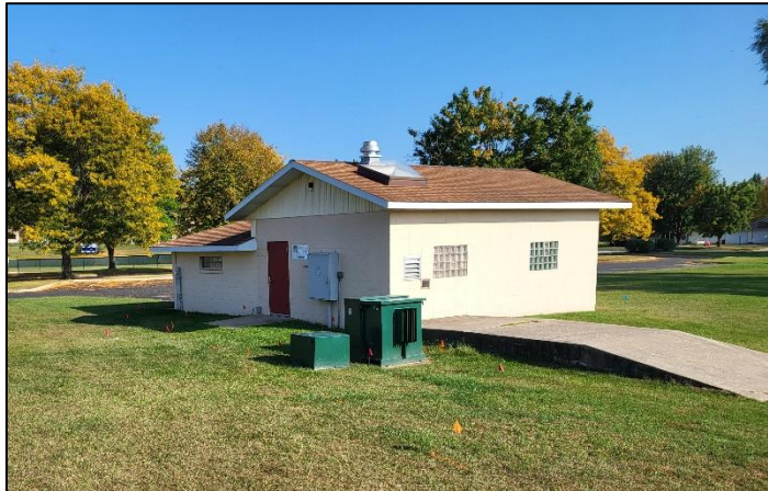
Wellhouse #6: Looking Southeast
