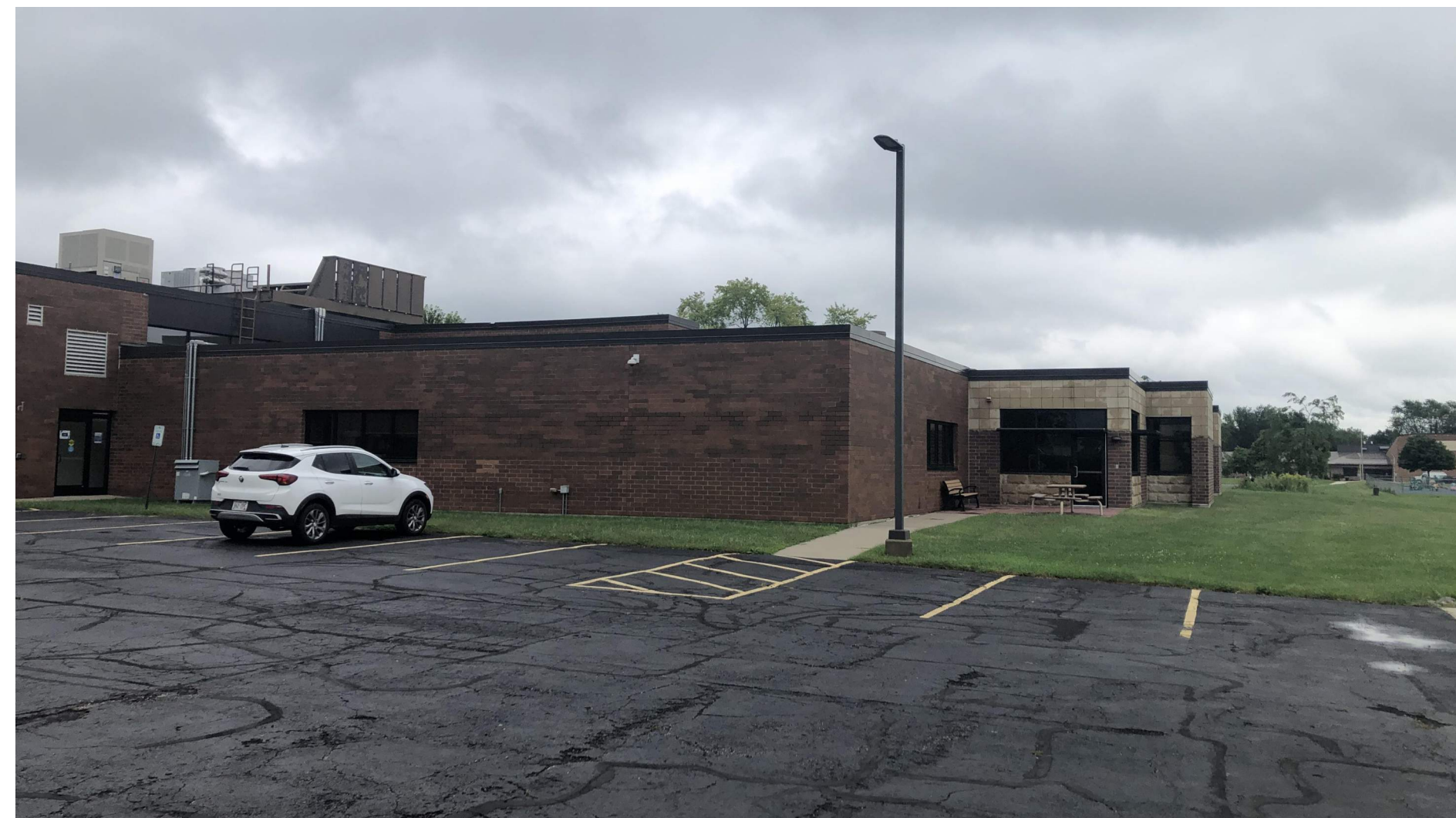
IMAGE 1 EXISTING BUILDING - WEST FACADE
