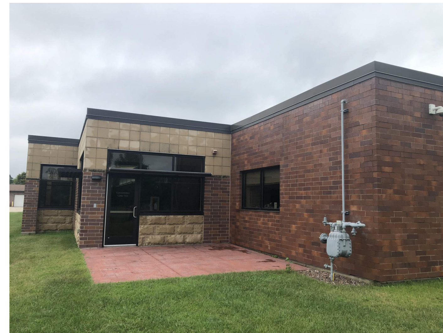
IMAGE 3 EXISTING BUILDING - EAST FACADE
