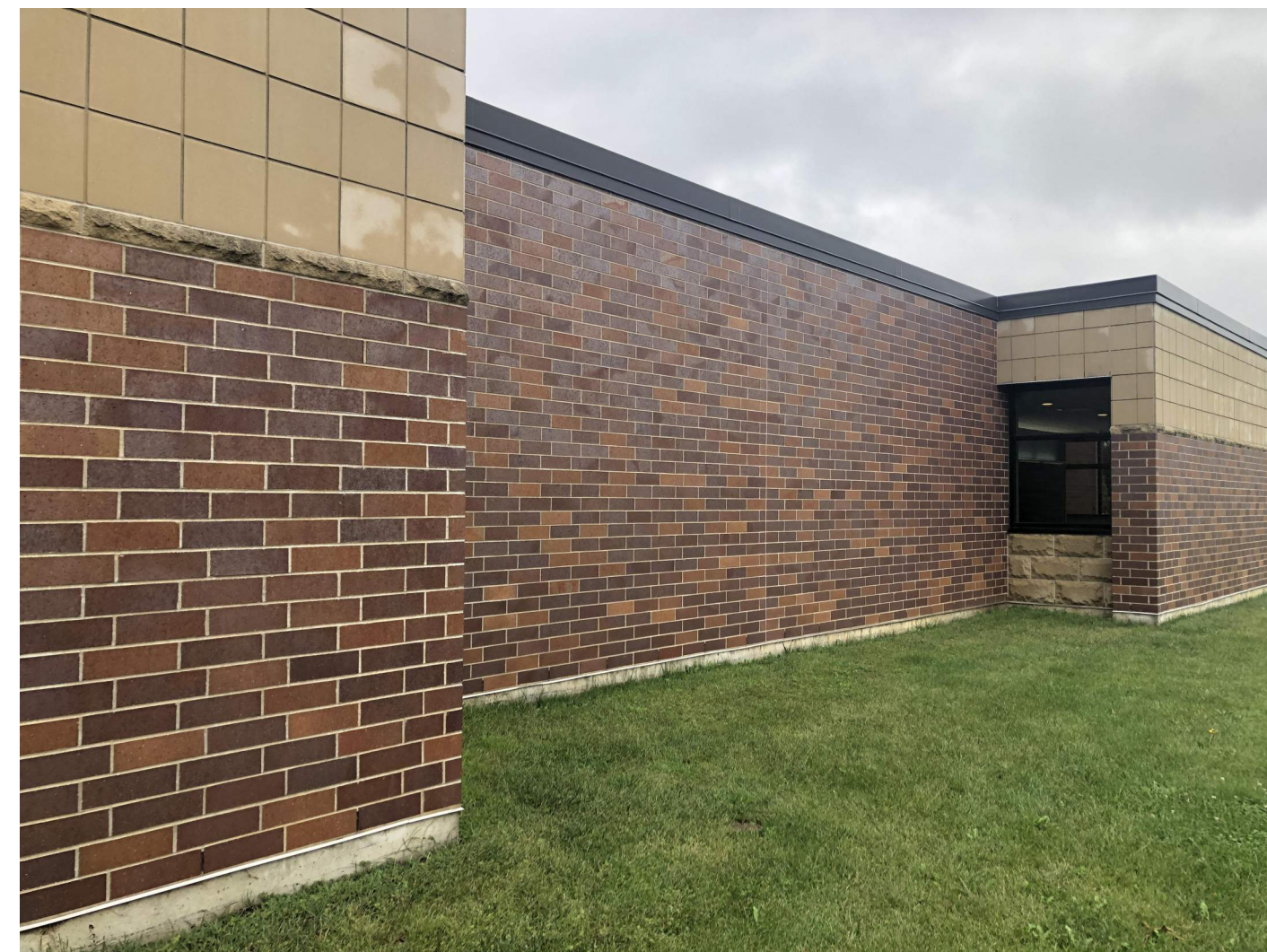
IMAGE 2 EXISTING BUILDING - SOUTH FACADE
