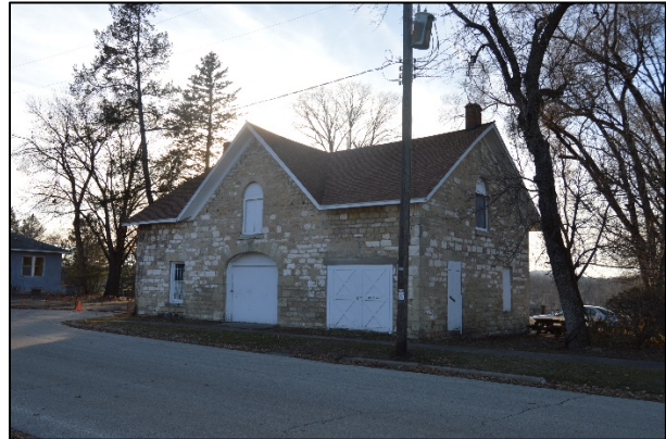
Service building (c.1860), 425 S. Prairie Street.
