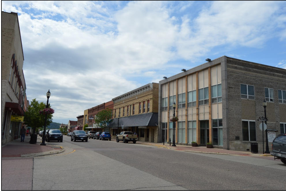
100 Block of E. Blackhawk Avenue in proposed Blackhawk Avenue Commercial Historic District
