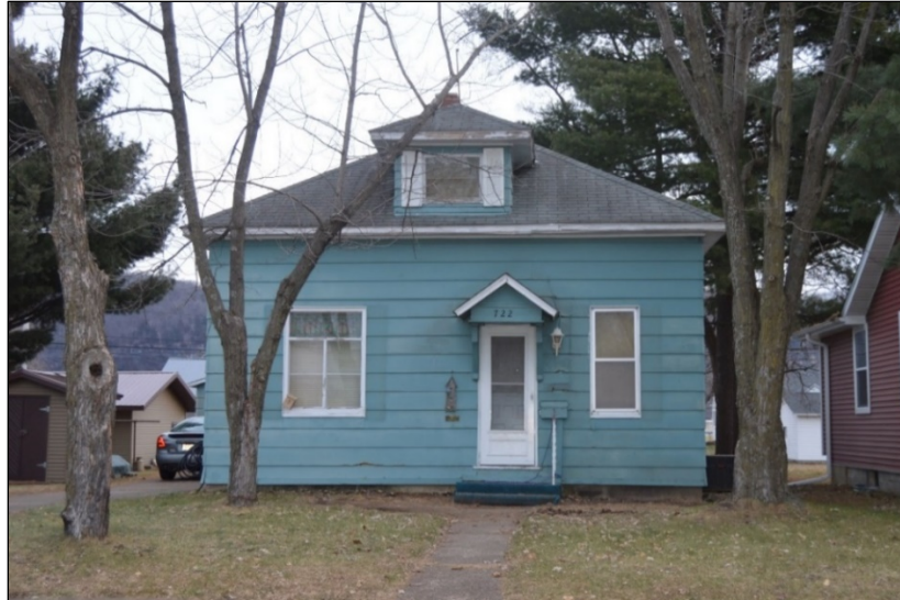
House (1912), 722 N. Beaumont Road
