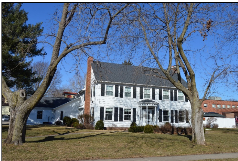
House (c.1925), 505 S. Michigan Street
