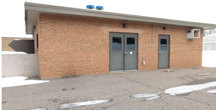
Original Blower Building
