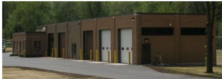
View of Administration Building / Garage from NE
