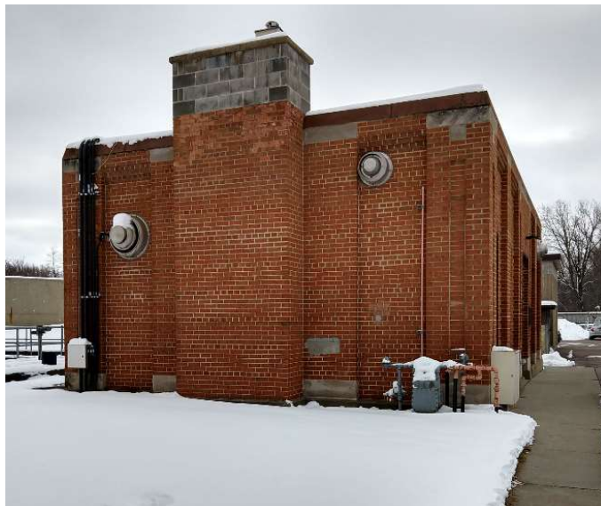
View of Control Building from South
