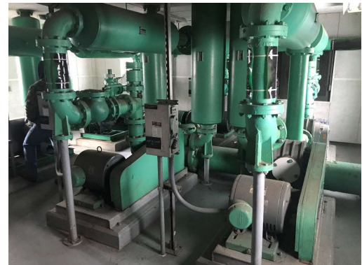
Blowers in Structure 36
