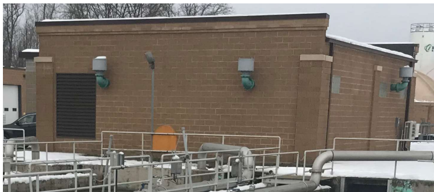
New Blower Building
