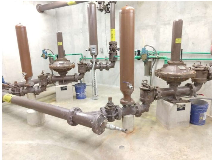
Air-Operated Diaphragm Pumps
