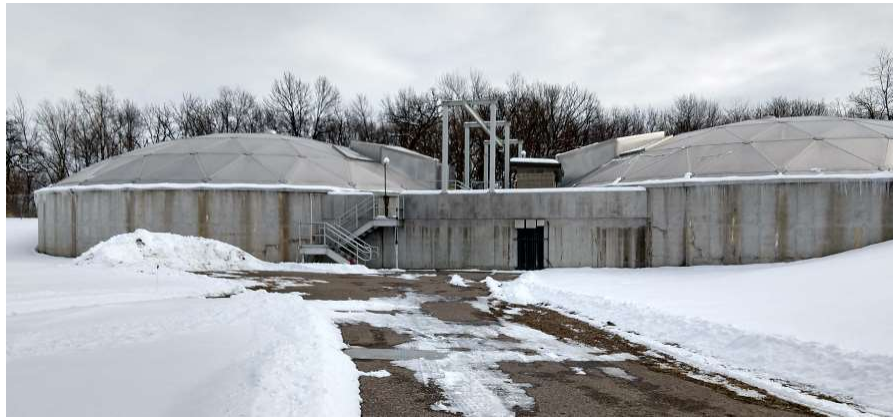
View from SW of Final Clarifiers
