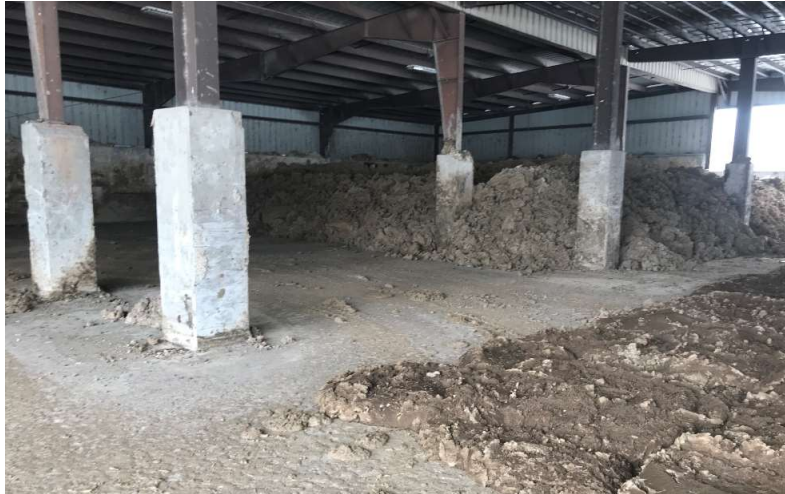
Inside Covered Sludge Storage Area
