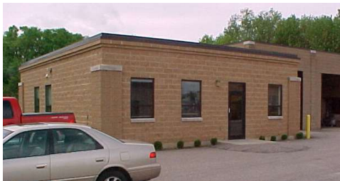
Front of Administration Building
