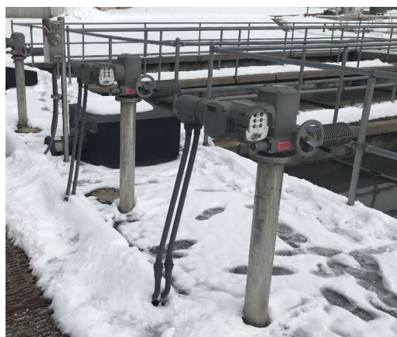
Electric Gate Actuators
