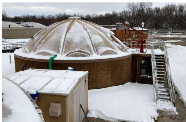
South Holding Tank & Blower Shed
