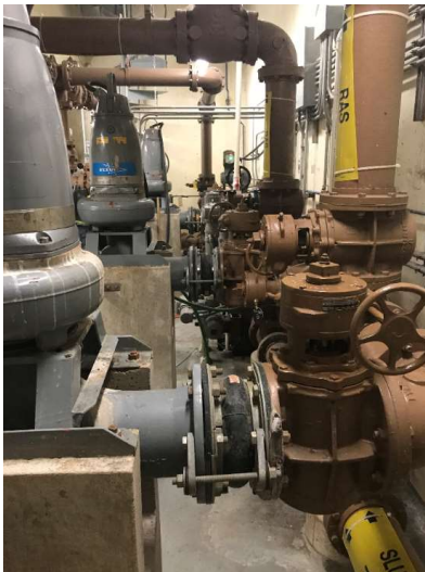
RAS Pumps/Piping/Valves
