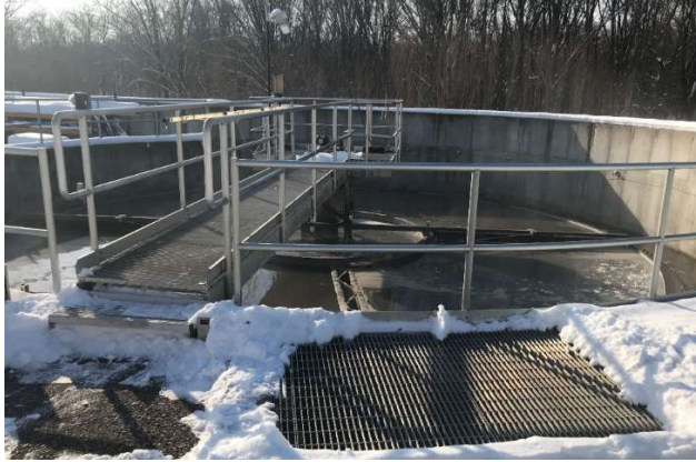
Exterior of Circular Primary Clarifier
