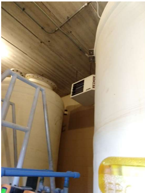
Inside Chemical Feed Building
