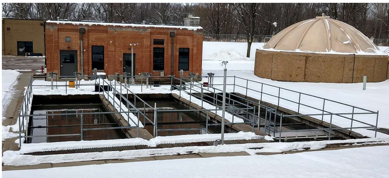
Rectangular Primary Clarifiers
