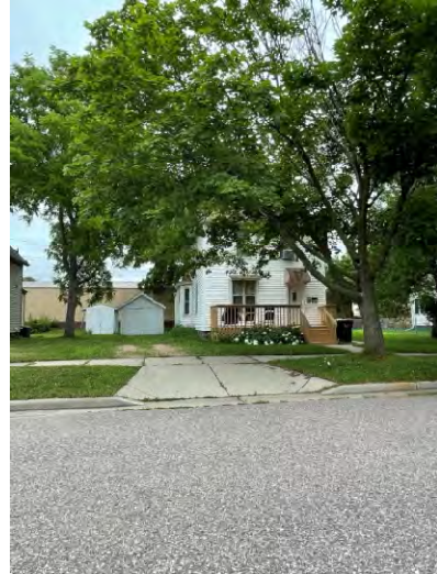
MAP ID 46 – Parcel 1649: 322 S. Locust Street. Lacking a driveway, deteriorating site improvements. Garage too small.
