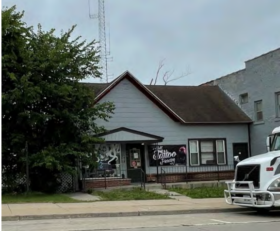
MAP ID 30 - Parcel 957-10000: 334 E. Main Street. Deteriorating site improvements, age of structure
