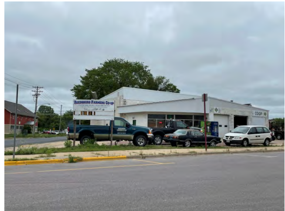
MAP ID 21 - Parcel 1007: 244 S. Walnut. Age of structure. Deteriorating structure and site improvements.
