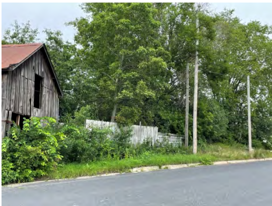
MAP ID 19 - Parcel 1005-10000: Rear of lot – deteriorating site improvements.
