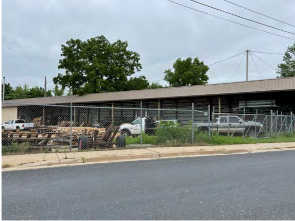
MAP ID 49 - Parcel 1652: 325 S. Park Street. Deteriorating site conditions. Obsolete platting.
