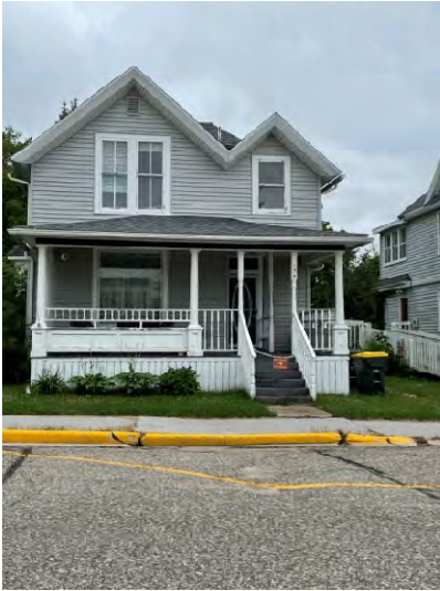
MAP ID 19 - Parcel 1005-10000: 156 Vine Street. Deteriorating structure and site improvements
