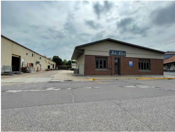
MAP ID 49 - Parcel 1652: See above. Façade view of address side of property.
