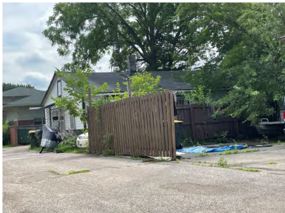
MAP ID 40 - Parcel 1037: 225 S. Park Street. Obsolete platting. Deteriorating site improvements.
