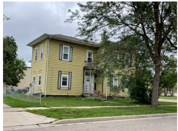
MAP ID 48 - Parcel 1651: 300 S. Locust Street. Deteriorating structure. Lack of a garage. Windows blocked.
