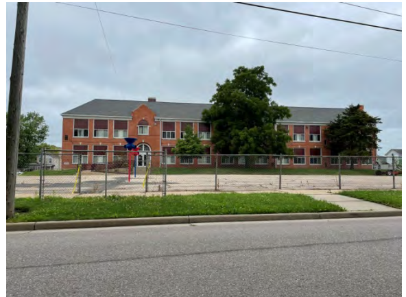
MAP ID 50 - Parcel 1640: 420 Plum Street. Deteriorating site improvements.
