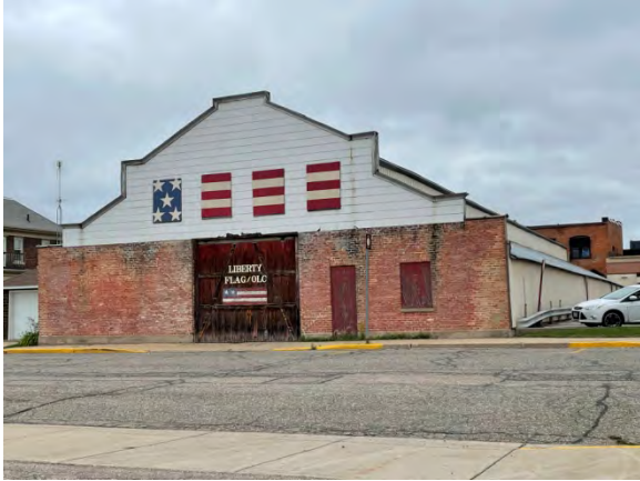
MAP ID 1 - Parcel 994: 121 S. Webb (view from Vine St.). Deteriorating site improvements, age of structure.
