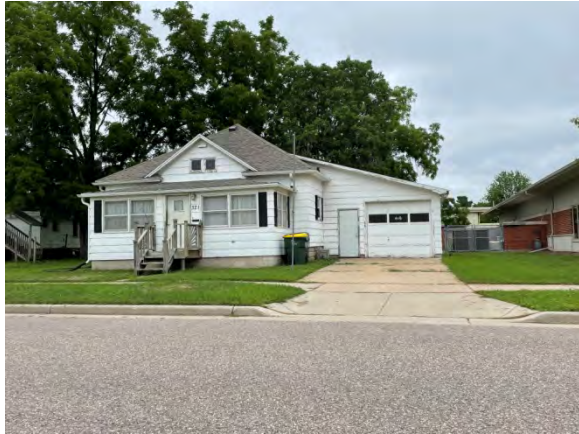
MAP ID 39 - Parcel 1036: 321 Plum Street. Old and deteriorating roof and structure.
