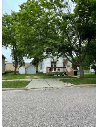
MAP ID 46 – Parcel 1649: 322 S. Locust Street. Lacking a driveway, deteriorating site improvements. Garage too small.
