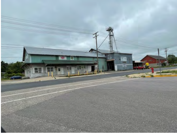
MAP ID 22 - Parcel 1008: Old and deteriorating structure.
