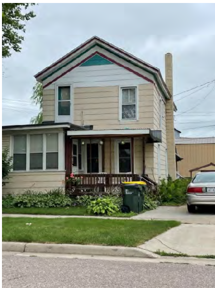
MAP ID 44 - Parcel 1647: 336 S. Locust Street. Garage too small. Deteriorating structure.
