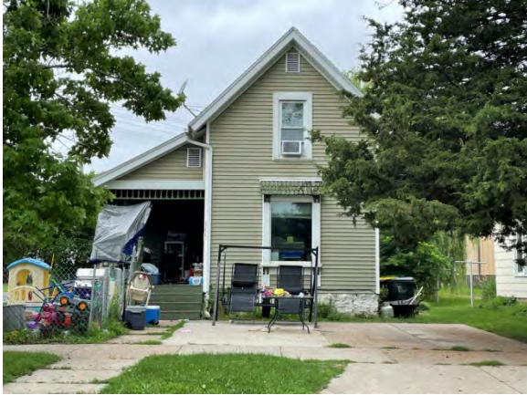
MAP ID 43 – Parcel 1646: 344 S. Locust Street. Obsolete platting, no garage.
