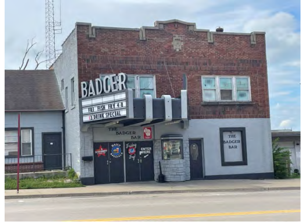
MAP ID 28 - Parcel 959: 326 E. Main Street. Deteriorating structure and age of structure.
