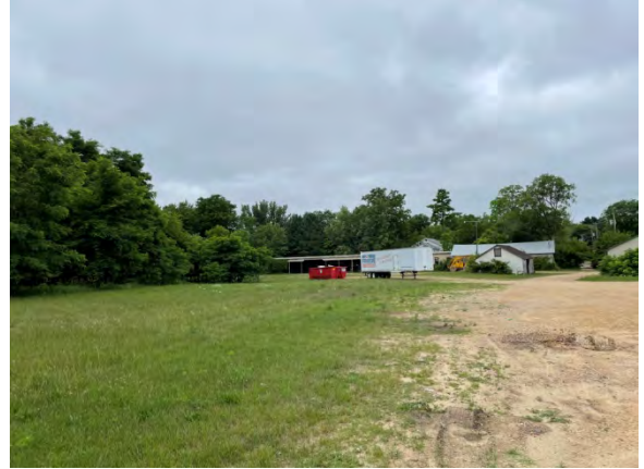
MAP ID 55 - Parcel 481: 410 South Avenue. Deteriorating buildings that are old and obsolete. Site improvements are deteriorating.
