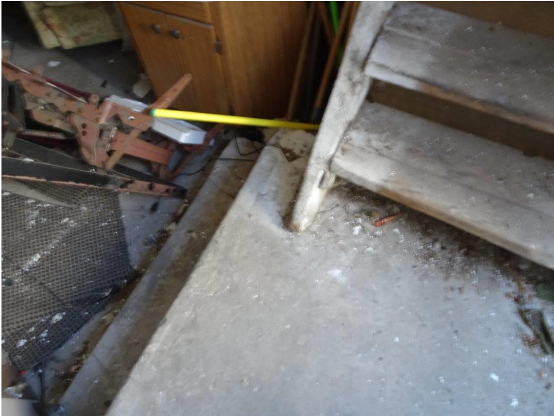
Photo 4.2.5 – First Floor Interior Step Down from Grade
