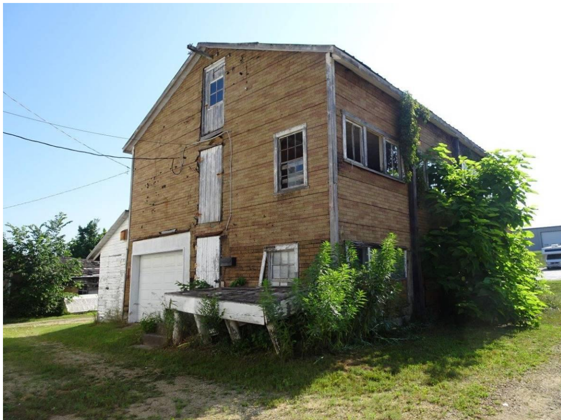
Photo 4.2.2 – Storage Building Exterior View South-West
