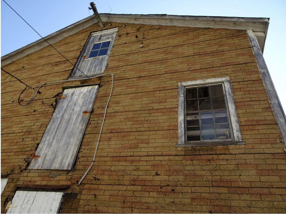
4.2.15 – Second Floor and Attic / Loft Level Doors Swinging to Exterior Open Air
