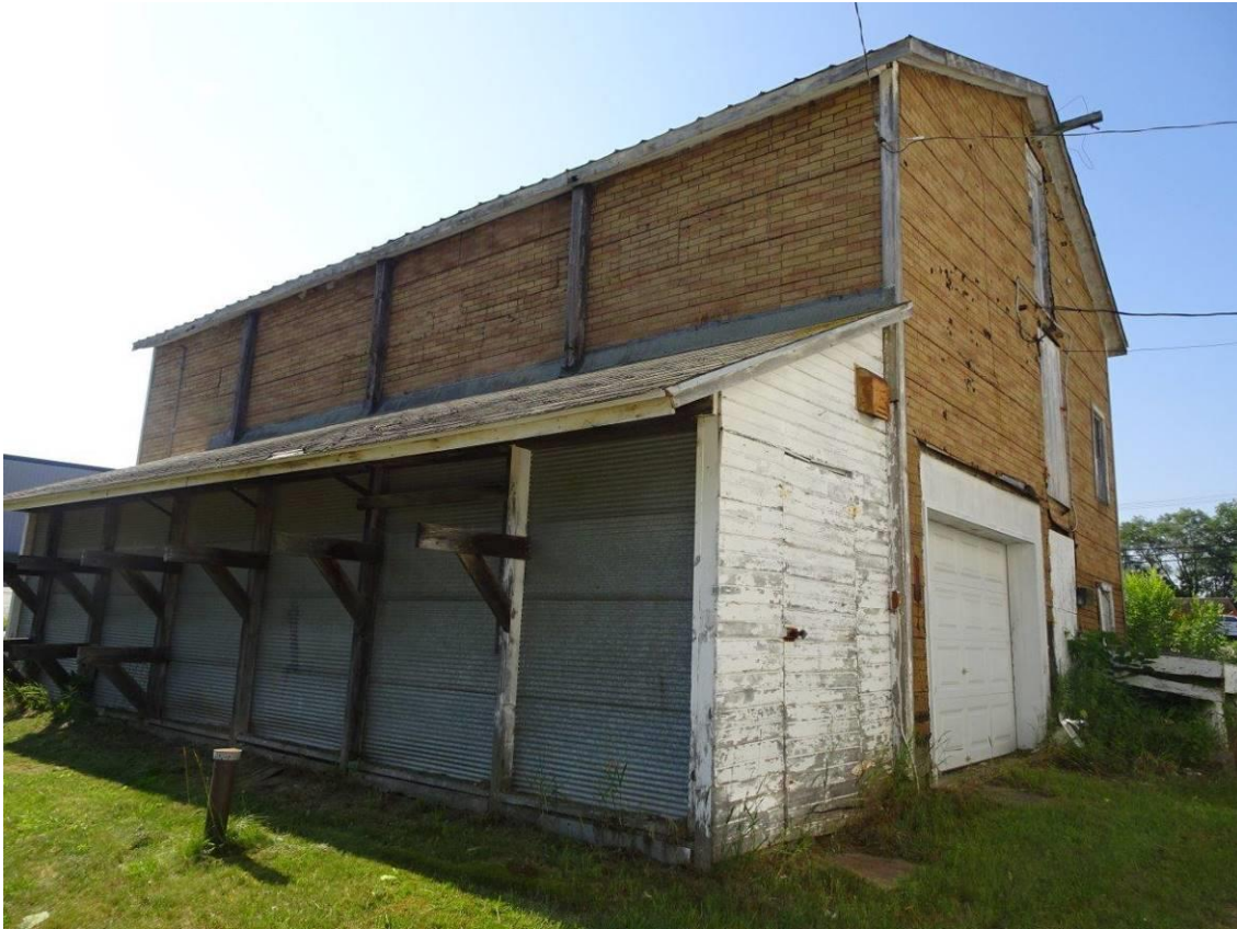
Photo 4.2.3 – Storage Building Exterior View North-West
