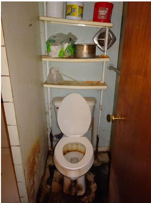
Photos 4.1.22 & 4.2.23 – Saturated and Rotting Bathroom Floor with Wall Mold
