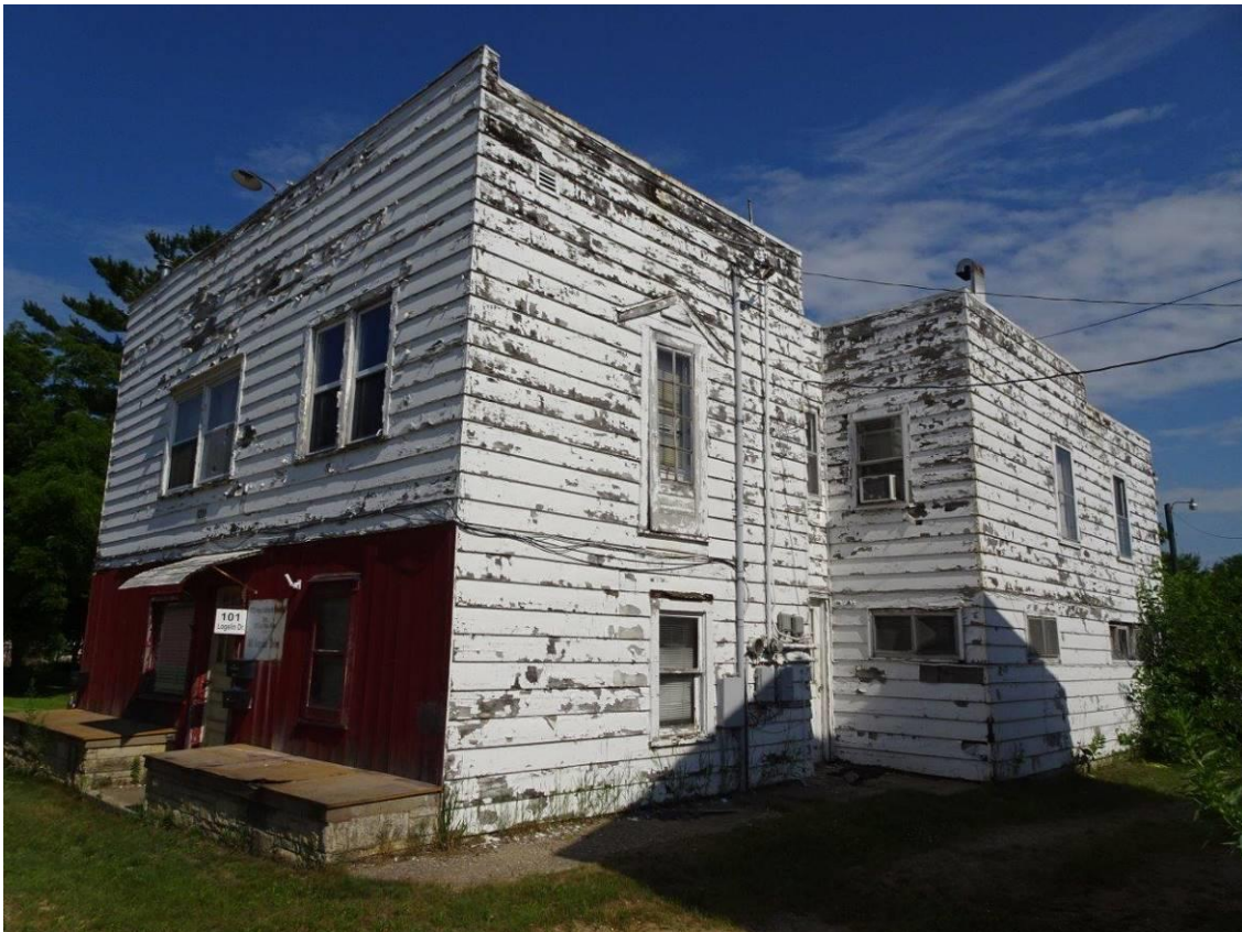
Photo 4.1.2 – Apartment Building Exterior View South-East
