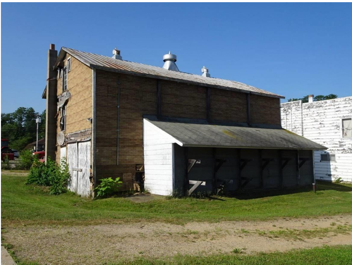
Photo 4.2.4 – Storage Building Exterior View North-East
