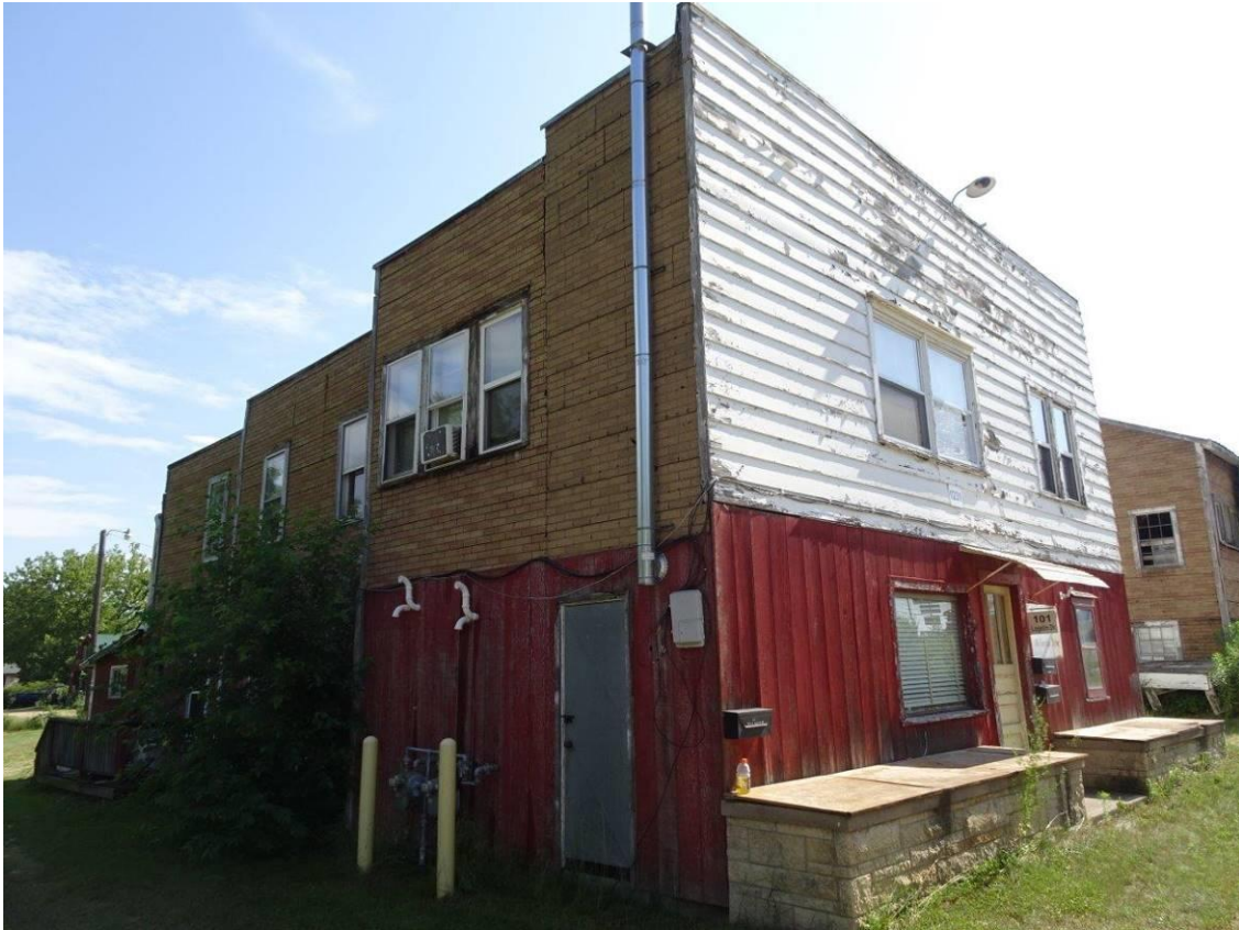
Photo 4.1.1 – Apartment Building Exterior View South-West
