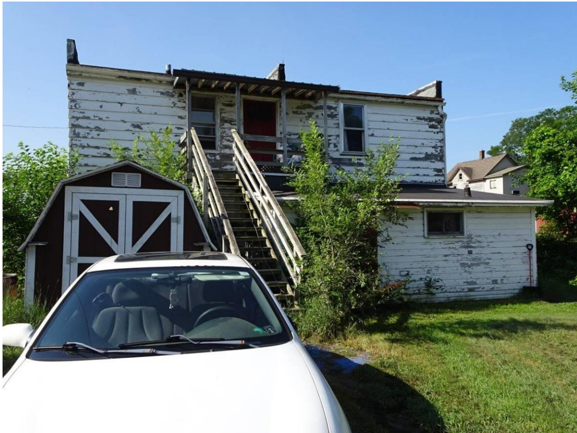
Photo 4.1.3 – Apartment Building Exterior View North-East
