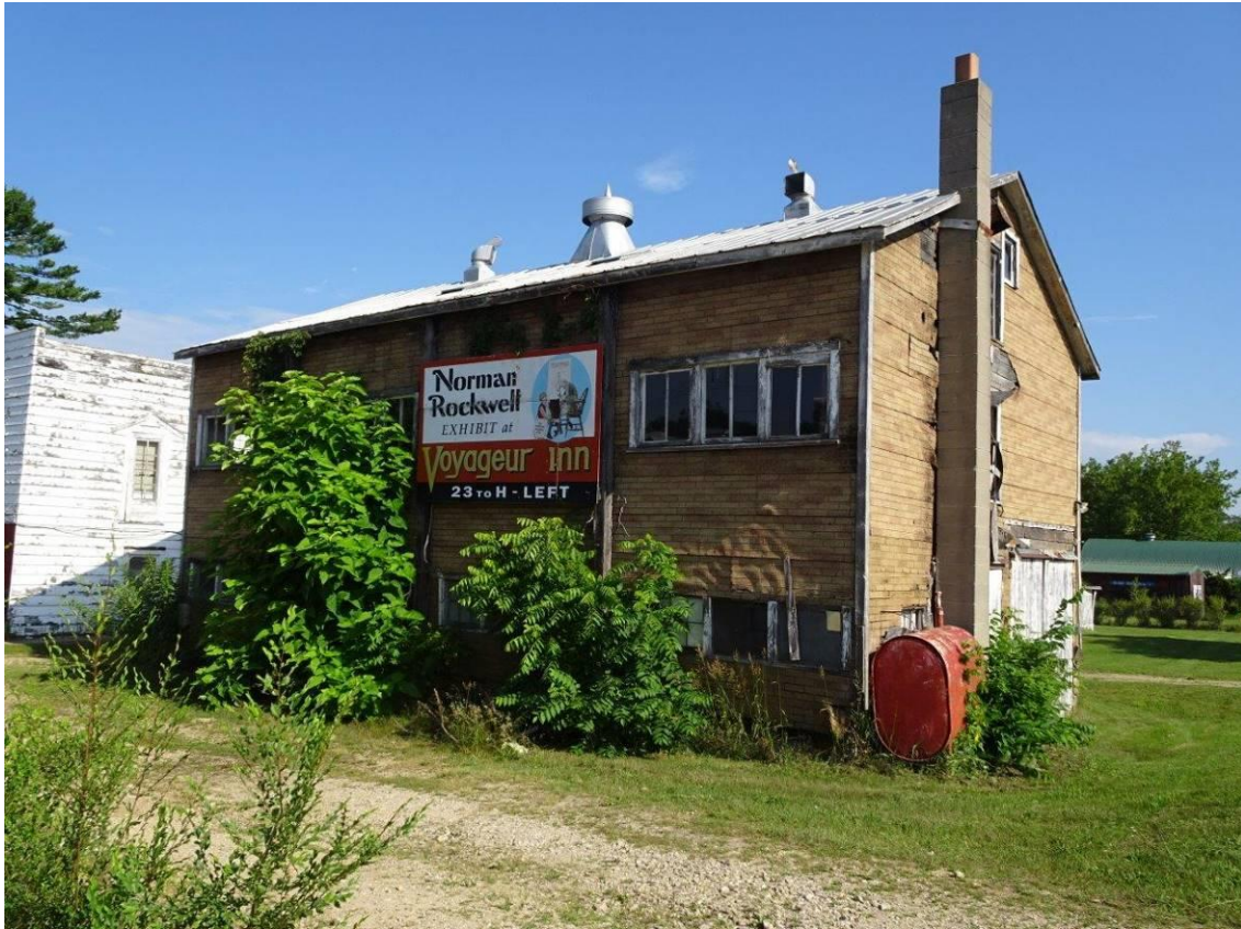
Photo 4.2.1 – Storage Building Exterior View South-East
